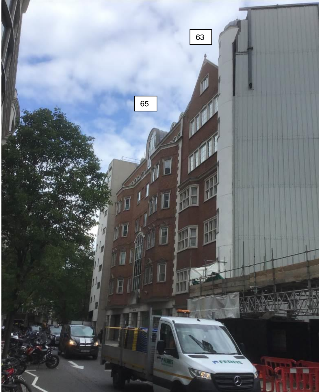
Curzon Street frontage
